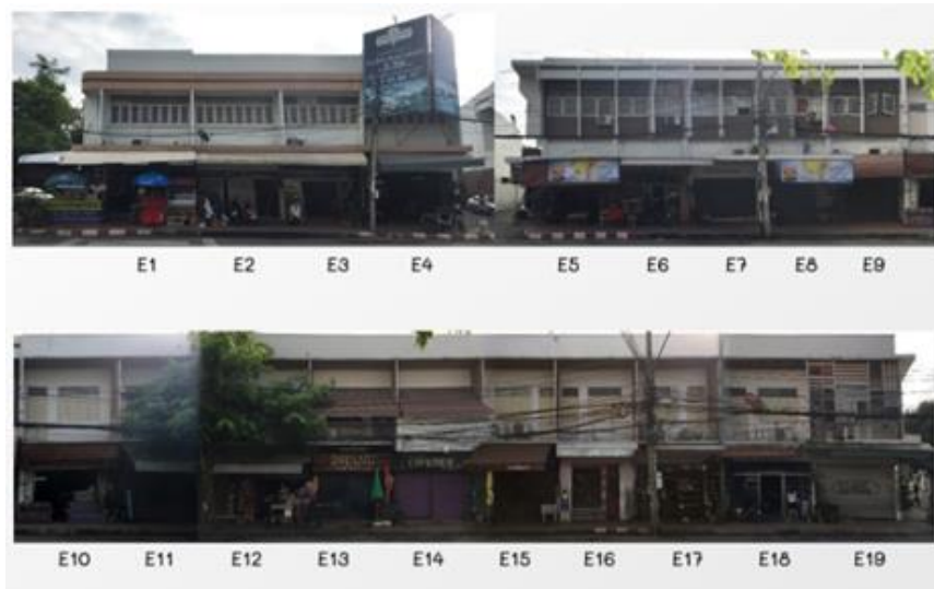
Fig.8 Building E1 – E19 of the East side
